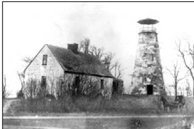
Barcelona Lighthouse, Lake Erie - first lighthouse to be illuminated by natural gas.
